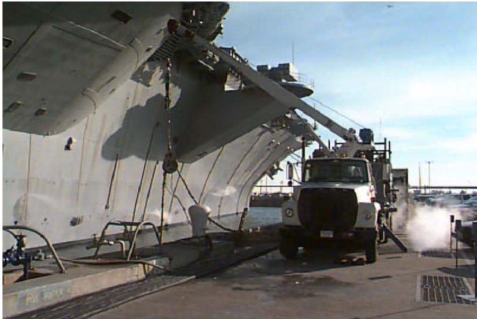
Figure 13-16. Cable Being Reeled by a Boom Truck.
