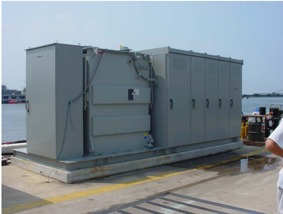
Figure 13-5. Skid-Mounted Substation with Single-Pole Connections
