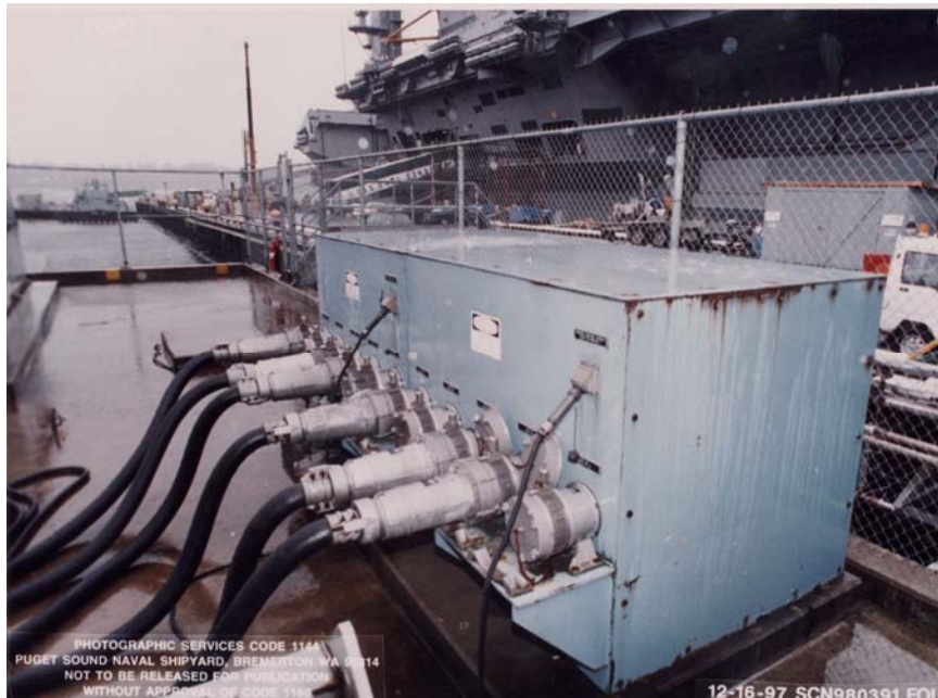
Figure 13-8. 4.16 kV Pier Electrical Outlet Assembly and Outlets
