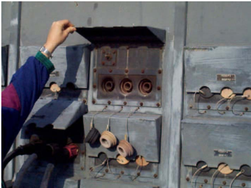
Figure 13-5. Skid-Mounted Substation with Single-Pole Connections
